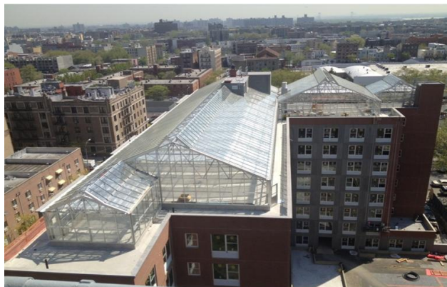
Fig. 1. Arbor House, New York, building with a greenhouse on the roof from the 1930s
