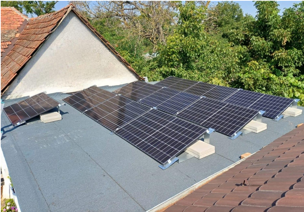
Fig. 2. Photovoltaic monocrystalline Canadian Solar 410W panel.
