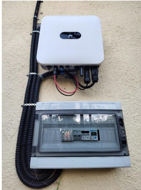
Fig. 3. Huawei Solar SUN2000-450W inverter
