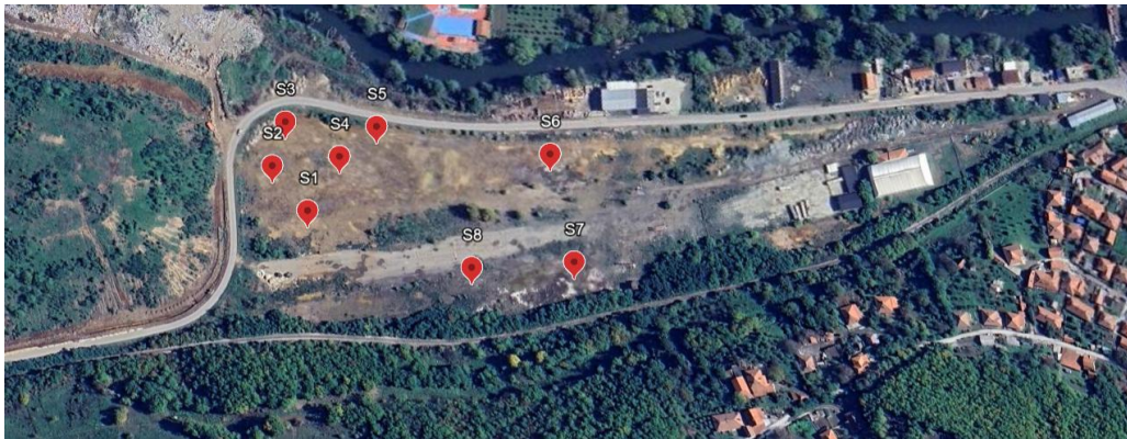
Fig. 2. Industrial waste deposit with sampling spots
