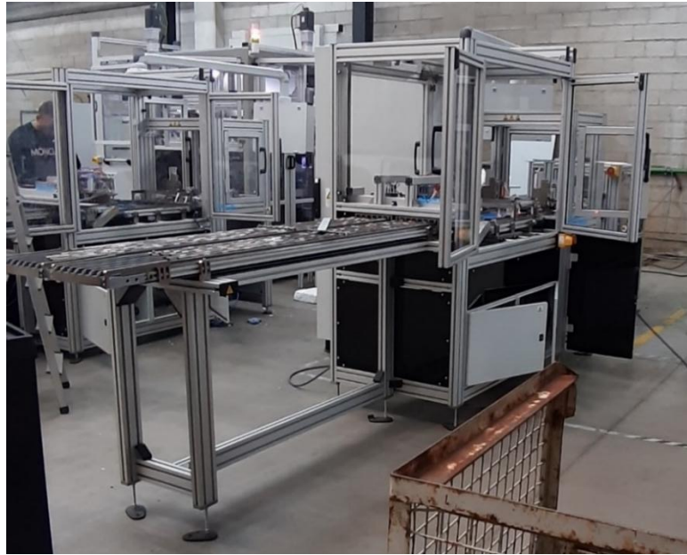
Fig. 3. Industrial control system from Experio d.o.o.
